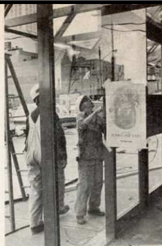
WORK PROCEEDS AT THE CITADEL Not a luxury, but a necessity.
